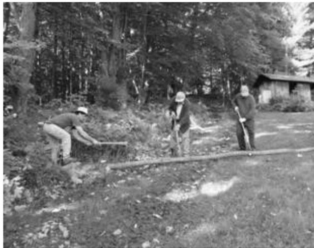
Volunteers install the first of 3 waterbars to divert water running down a tractor road in Montoomerv
